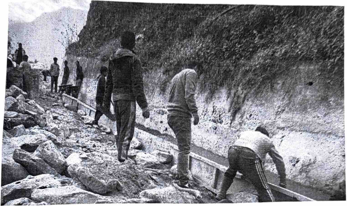
Monitoring on material mix and quality of work
