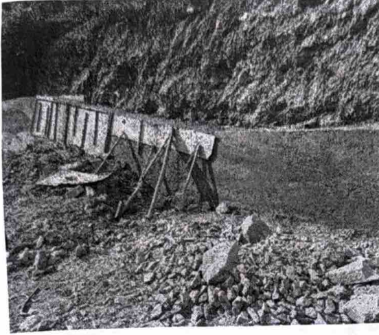
Formwork Placement of Concrete retaining structure
